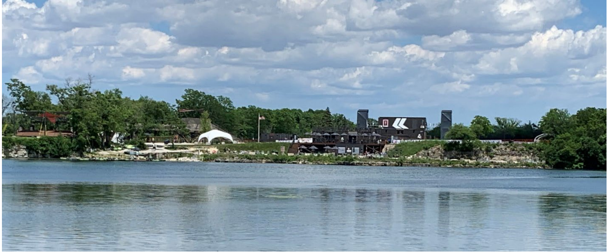
Figure 3: The Forge site, looking east from the west shore
